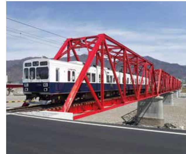
Restoration of the Chikuma River Bridge
