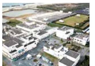
Hamamatsu City Public Wastewater Treatment Plant (Seien Area) Management Project (Courtesy of Veolia Japan)
