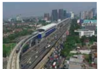
Jakarta Mass Rapid Transit (MRT) project, CP 101 and CP 102 areas (Indonesia)
